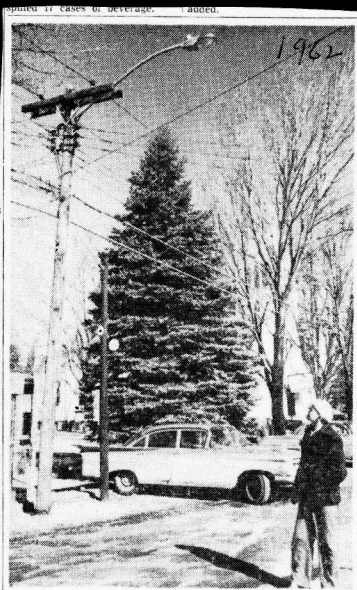
NEW STREET LIGHT — Kenneth Mullins of Pine Island observes new street light near St. Stanislaus Church, Pine Island. Sixty-five new street lights will be installed in Pine Island, Little York, Little Brooklyn and Edenville areas.
